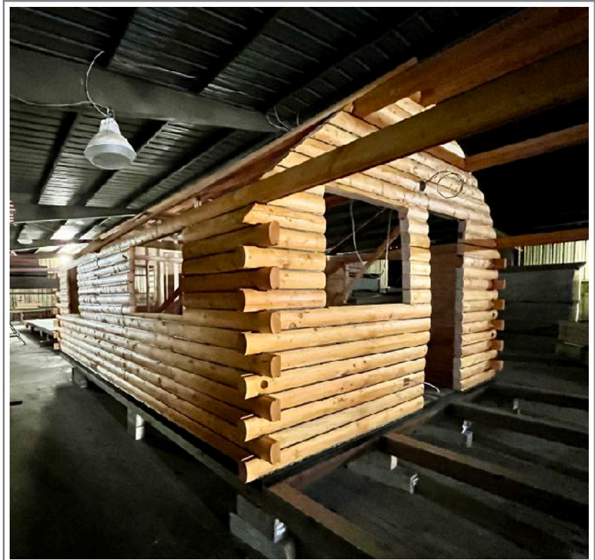
LIKE THE COTTAGE THE CABINS WILL BE BUILT IN GREAT FALLS AND TRANSPORTED TO CAMP
