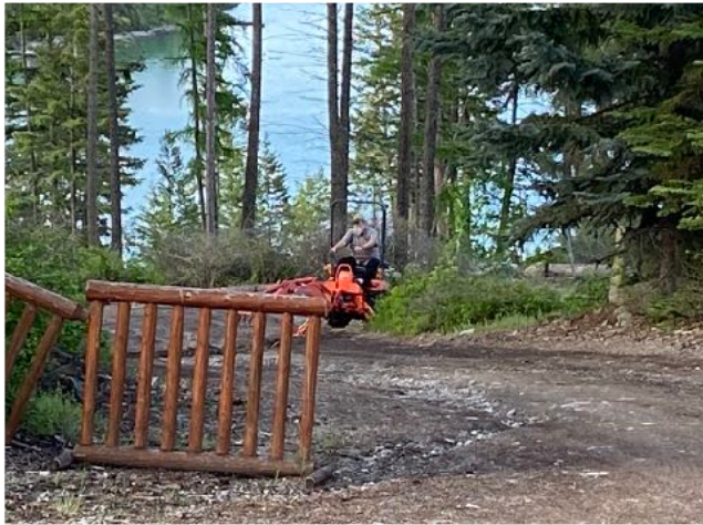
DON WORKING WITH HIS BACKHOE
